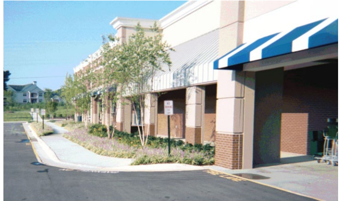
Example of Foundation Landscaping
